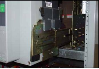
Figure 28. Switching Device in the REMOVE Position.
